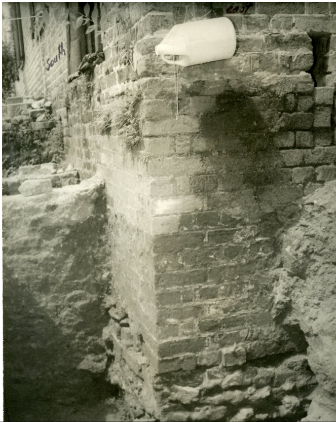
Figure 4: Kitchen foundation exposed during excavation sits on earlier brick feature.
